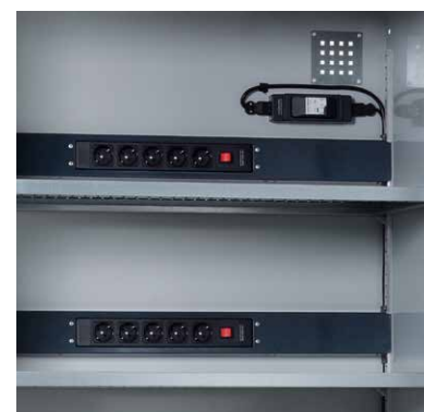
Rear panel installation
