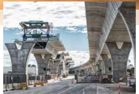
Structural and civil engineering
